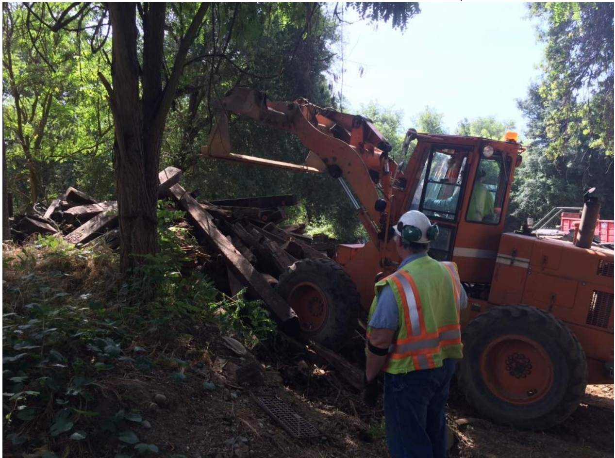
Frank digs-in to the dead tie pile. Aren't big machines great?
